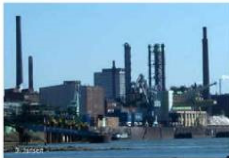
heating systems manufacturers
